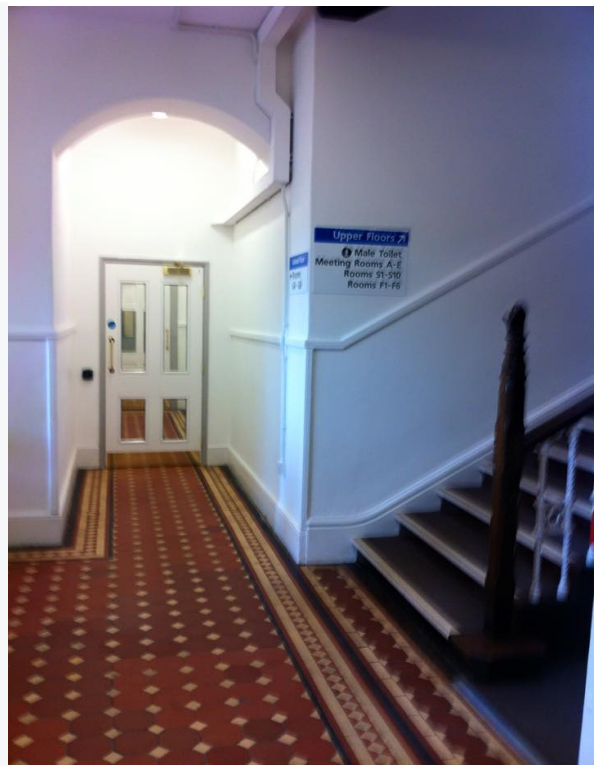
New (note stair safety edges!)
